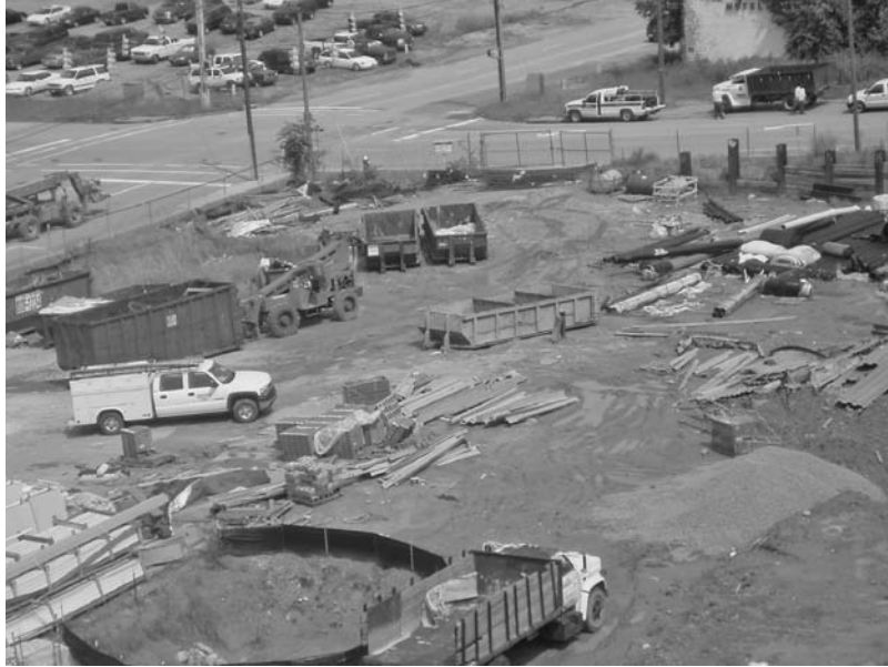
FIGURE 1.1.1 Construction debris container yard at a LEED registered project in 2005 at the University of South Carolina in Columbia, S.C. (Photograph taken by Steve Bruner.)
