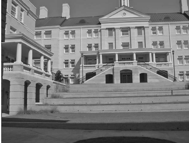
FIGURE 1.1.2 Landscaped amphitheater also functions as a stormwater management feature at the LEED Certified West Quad Housing Complex at the University of South Carolina. (Photograph taken in September 2006.)
